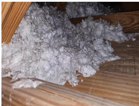
2330-2 Insulation Typical Interior
