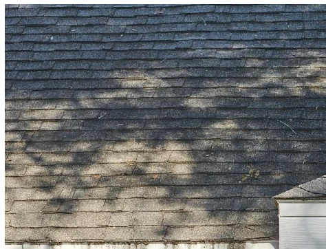
2330-3 Asphalt Shingle/Tar Typical Exterior Roof
