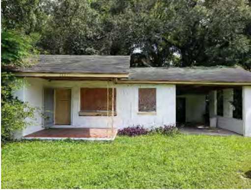
Exterior South Wall
