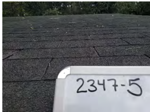
2347-5 Asphalt Shingle Exterior Roof
